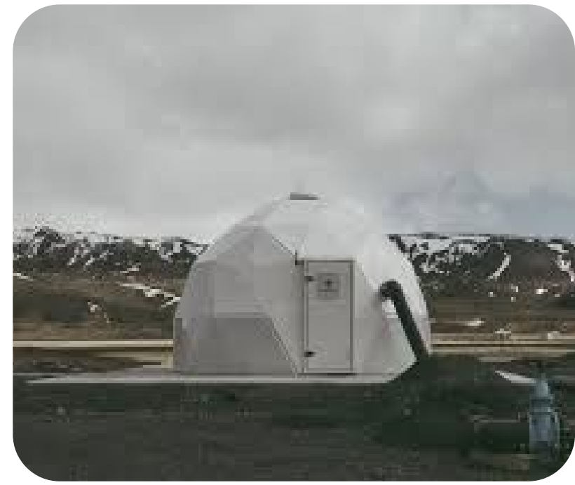
Injection well or igloo where CO_2 is permanently sequestered.
